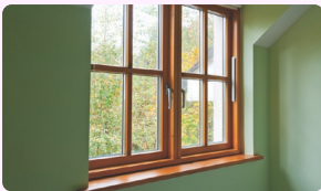
Window & Window Frame
